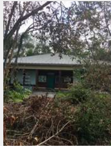
Castellow Hammock after Hurricane Irma. Courtesy of Linda Evans
