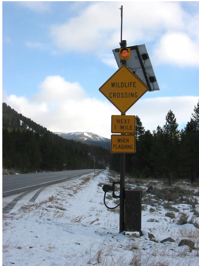
Figure 2: Experimental roadside animal detection – driver warning system in Yellowstone National Park (Credit: Marcel Huijser, WTI)
